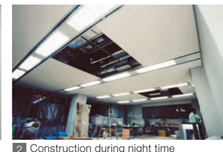
2 Construction during night time
