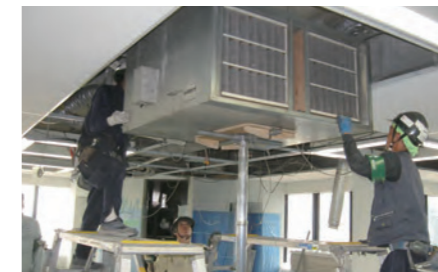
2 Removing existing indoor unit
