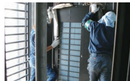
7 Outdoor unit installation
