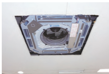
New indoor unit installed
