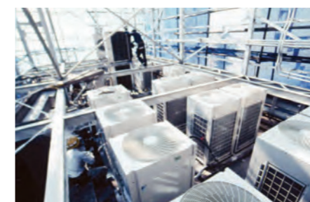
Replacement in progress
