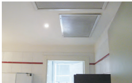
Installation was carried out during weekends to minimize disruption to business.
