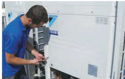
Thirty-nine VRV III-Q units serve 215 cassette type indoor units and 35 VAM ventilation units.
