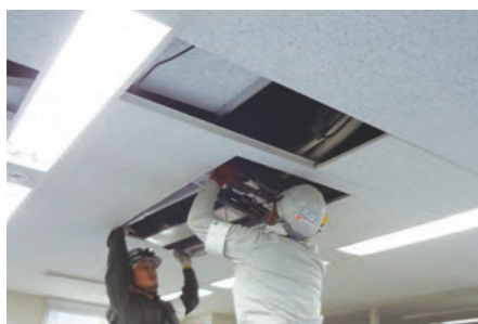
Removing old indoor unit
